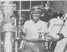
A PROBE-type sample connection for product lines is positioned by J. C. Walker, assistant shift foreman in Process-Cracking and Light Ends. Its use was suggested by Mr. Walker who was awarded a Fls. 700 CYI award in August. His idea was also named the CYI-of-the-Month. MUESTRA DI un conexion pa sonda muestra ta worde posisioná door di J. C. Walker, assistant shift foreman den Process-Cracking & Light Ends. Su uso a worde sugeri door di Sr. Walker kende a gana Fls. 700 pa e idea aki na Augustus. E idea aki tabata e mého di Augustus.
